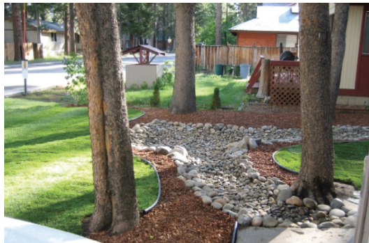
Figure 8: This infiltration basin will store roof runoff until it can percolate into the ground [3].
